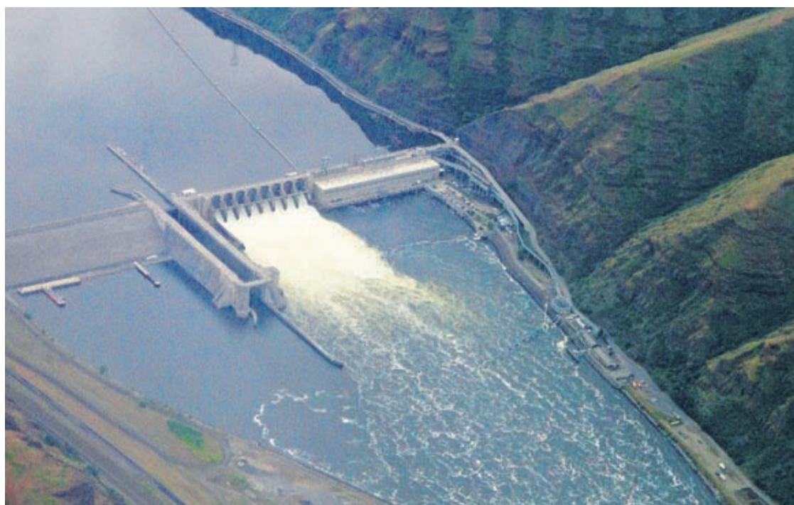
In this May 15, 2019 photo, the Lower Granite Dam on the Snake River is seen from the air near Colfax, Wash.
